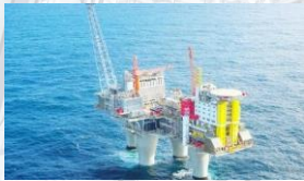
洋上への送電 Power from shore
