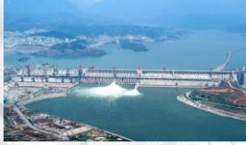
遠隔電源の送電 Connecting remote generation
