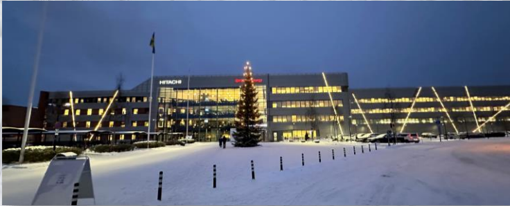
Uno Lamm HVDC Center, Hitachi Energy Ludvika
